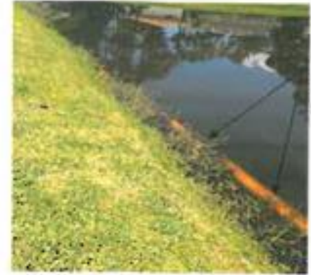
Exposed Underdrain pipe
